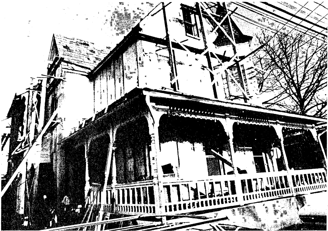
FIGURE 2.2 A grantee in Pennsylvania decided on an exterior retrofit of this historic structure so that the building tenants could remain in the house during construction. Photo credit: Rodale Press.
