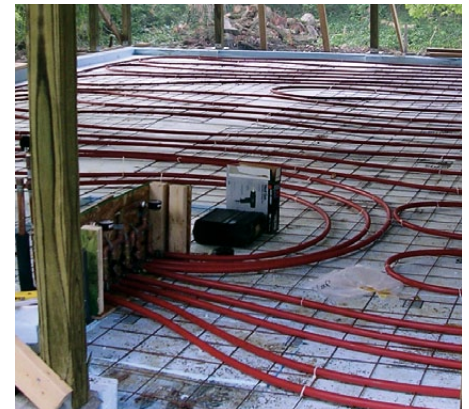
Bob’s house has radiant floor heat, under-slab insulation, and a solar hot water system for heating and domestic hot water.
