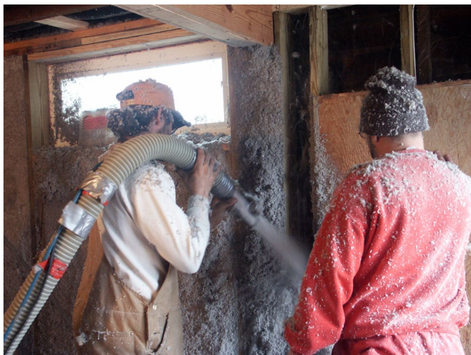
Wet cellulose insulation being blown into 12' thick walls for a Passive House retrofit.
