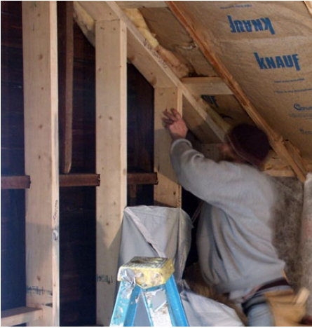
Adding double studs for a Passive House retrofit.
